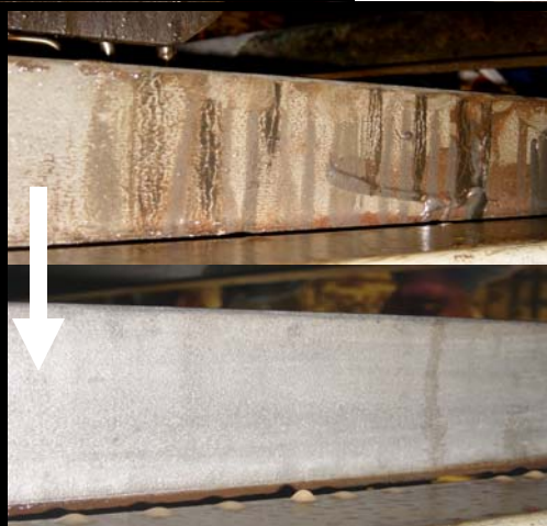
Removing chain grease and built up soils from cross beam (above) and drive sprocket (below)
