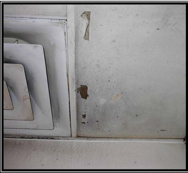
Ceiling tiles and T bars can be cleaned of dirt and oil using a suction tool which uses the vapor to penetrate pores and melt oils and suction to remove the soils and moisture leaving the surface dry.
